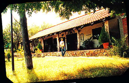
Laundry building and communal clothing room.
